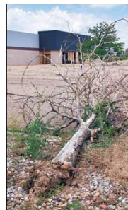
Abandoned Wal-Mart store on U.S. 50 in La Junta, Colorado has been vacant for four years
