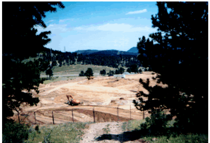
Construction on Clear Creek H.S., from Beaver Brook Canyon Rd.
